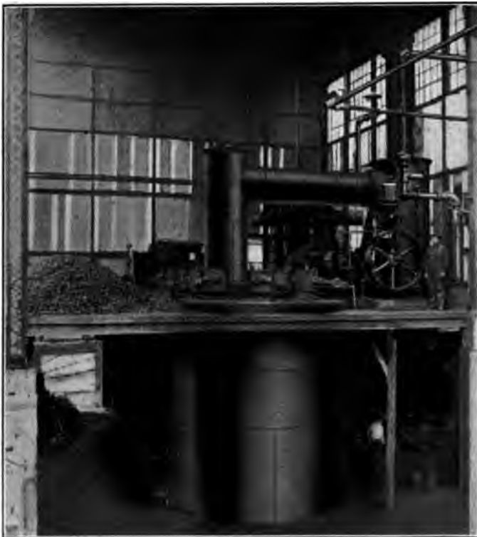
FIG. 231.—Smith gas producer plant.
